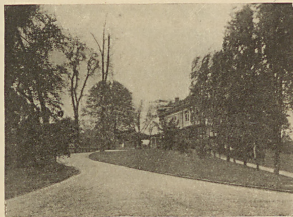
The house at Torresdale, with its garden views.
