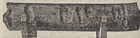
Electrolytically Pitted Water Pipe.
