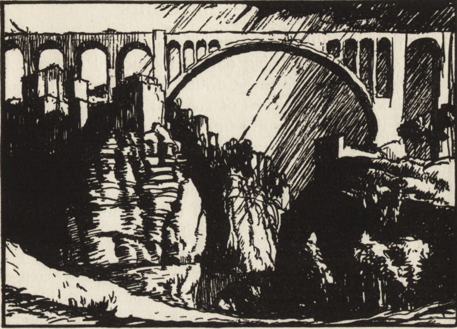
PONT SIDI RACHED AT CONSTANTINE, ALGERIA. BUILT IN 1908-1912
