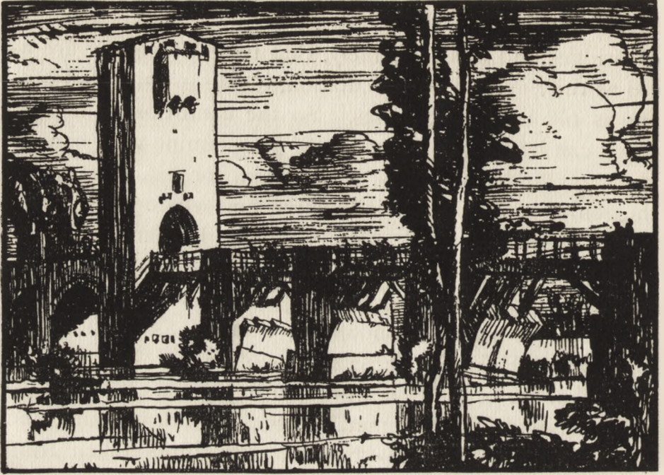
A BROKEN WAR-BRIDGE OF THE XIII CENTURY, AT NARNI IN ITALY ; REPAIRED WITH WOOD
